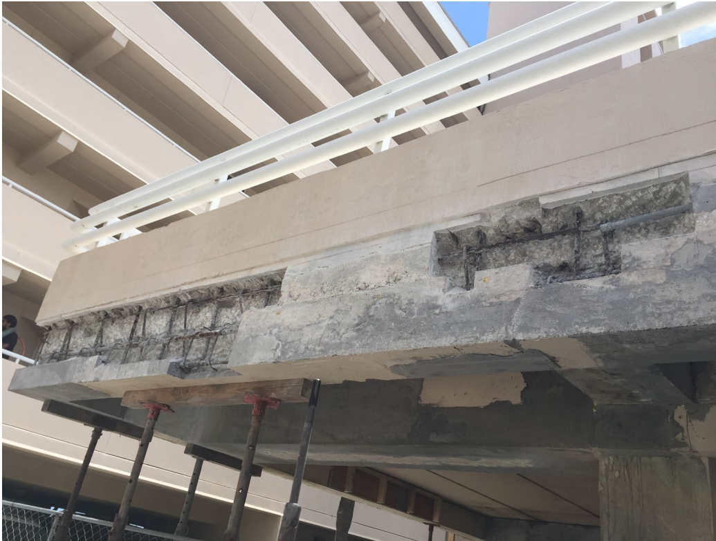
Picture 1: Completed excavations, not yet sandblasted
